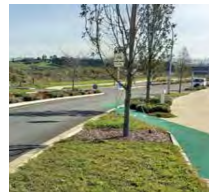
Taiatea Drive associated with Rotokauri Rise residential development
