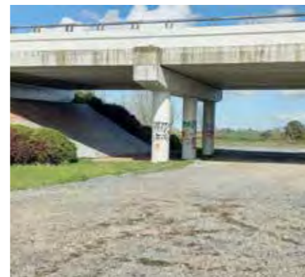
Chalmers Road underpass of Waikato Expressway
