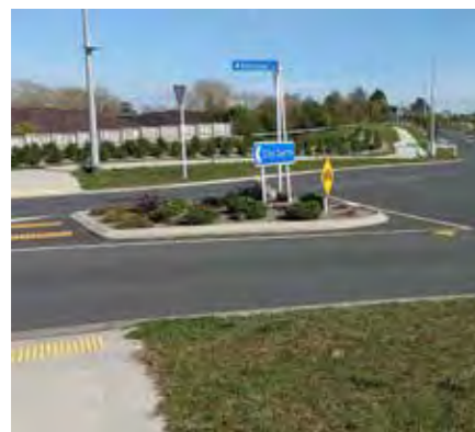
New roundabout with pedestrian island crossings and amenity planting on Rotokauri Road
